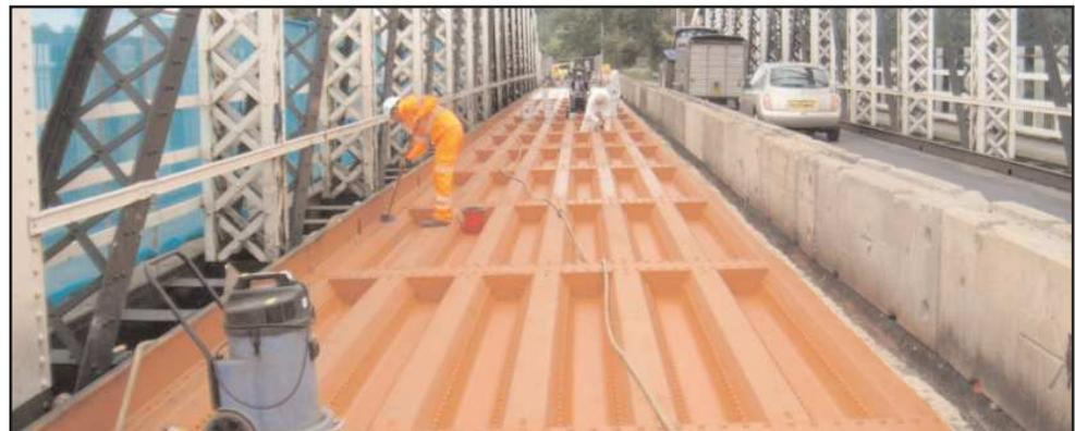
**A**cton Swing Bridge, on the River Weaver near Northwich, reopened on in July after a six month, £1.5 million programme to repair and strengthen the bridge deck.
